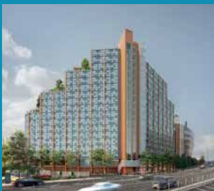
161 Talgarth Road - Under Construction
