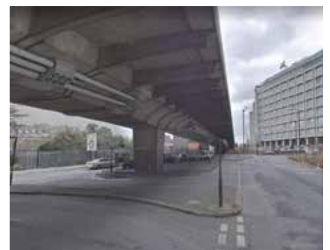
A4 Flyover looking west
