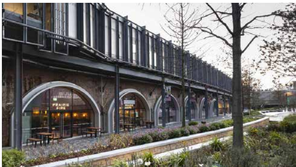
Renovated Railway Arches - White city
